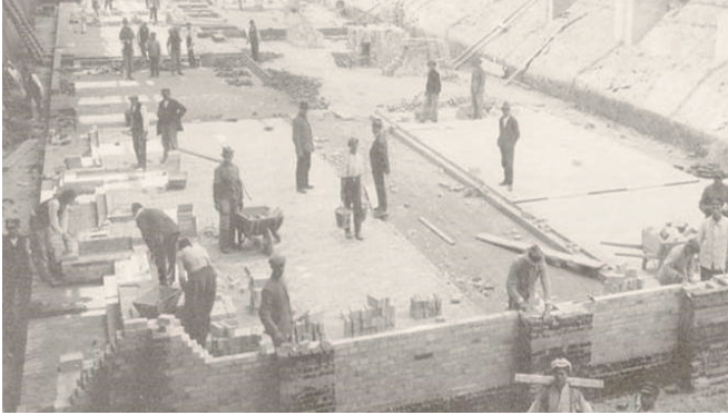
First Riedhammer Baking Furnace
